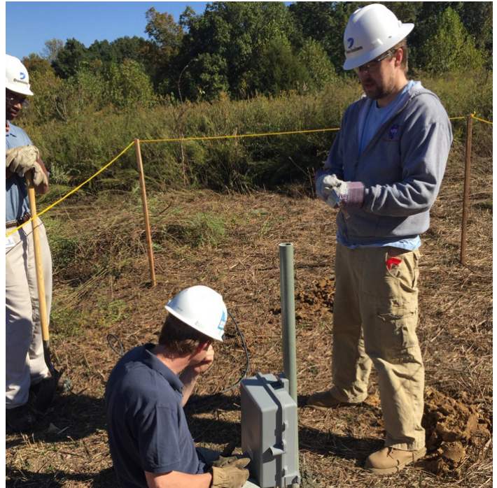
Goddard engineers and scientists installing scientific substations beneath high-power transmission lines. Photo Credit: GSFC
